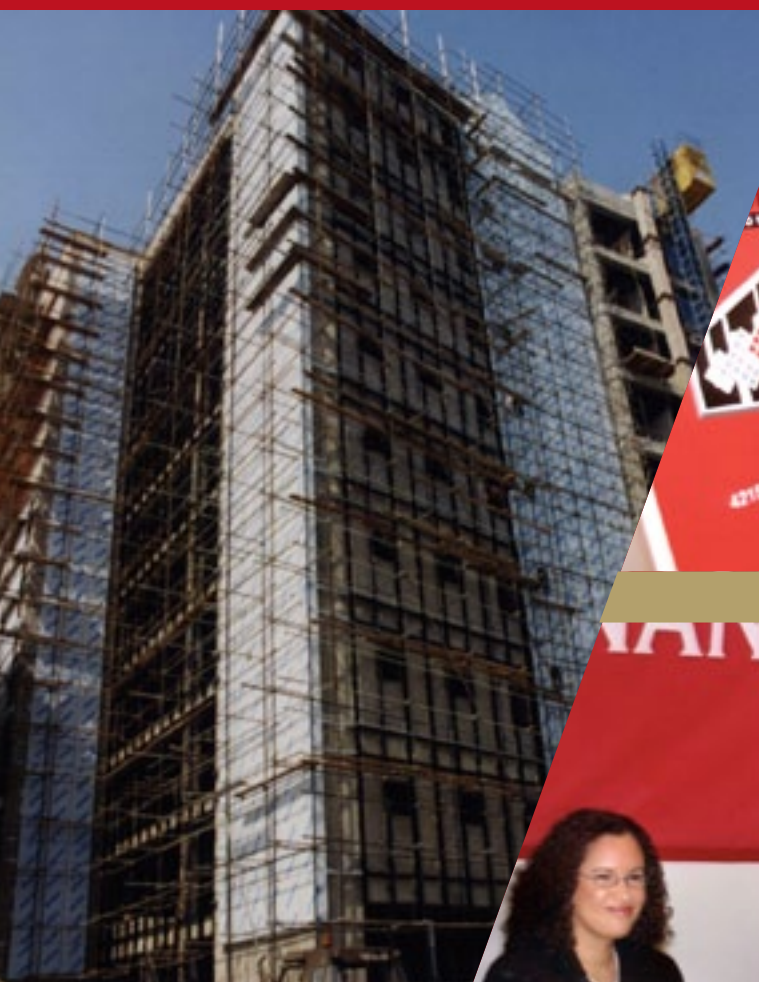
UTC Financial Centre in Port-of-Spain under construction
